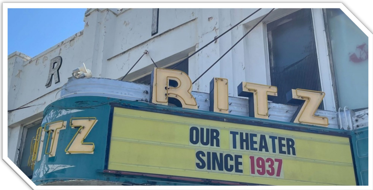
Ritz Theater Renovation
