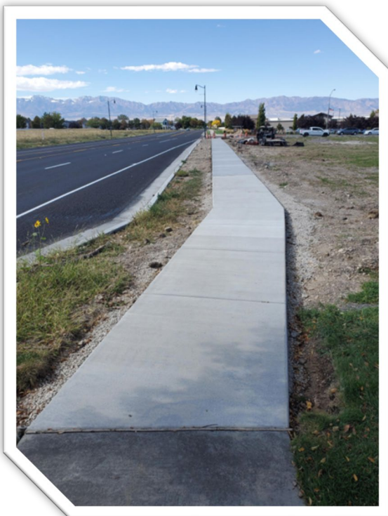
New Sidewalk along 2000 North
